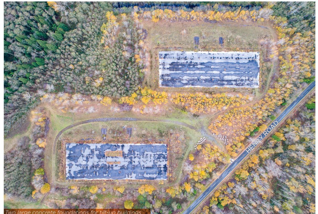
Two large concrete foundations for tilt-up buildings
